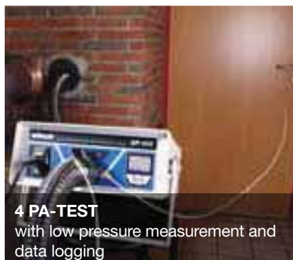
TIGHTNESS TESTING of all flue gas systems
